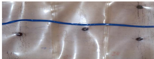
Installed Injection Hose spot welded to the Geomembrane
