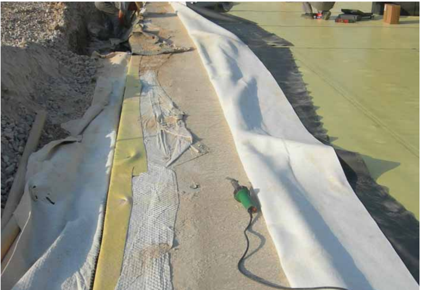
Connection Wall Ceiling Slab With working space
