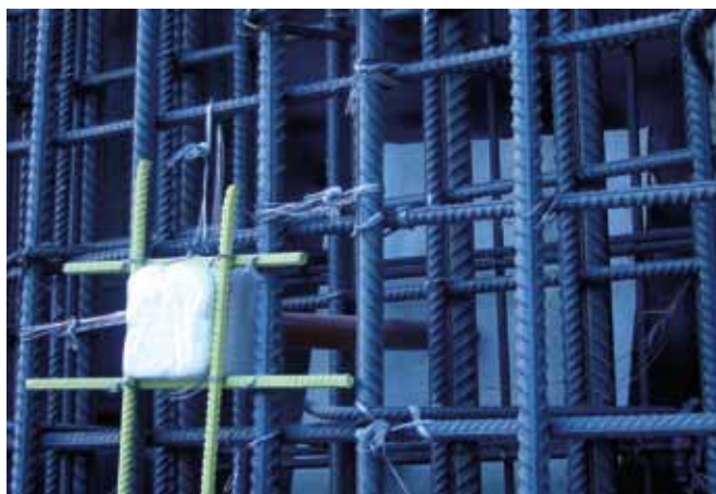
Protected inlet of Injection Pipe
