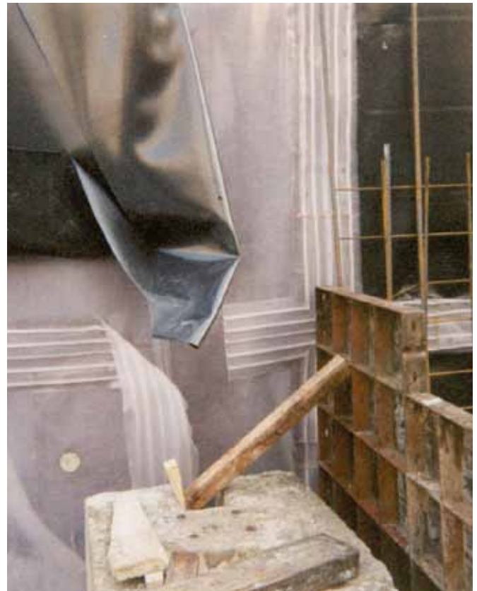
Water stop installed
