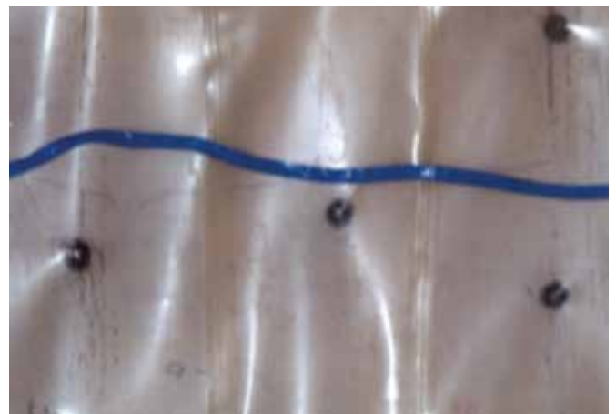
Injection tube welded to geomembrane
