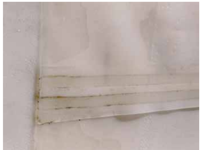
Double seam welding with translucent geomembrane
